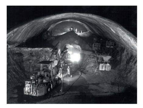
Fig1. Excavation of the experimental halls of the Gran Sasso Underground Lab.
