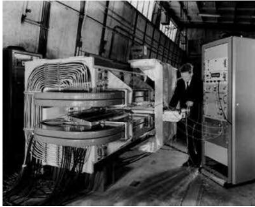
Fig. 3. Combined-function magnet in the process of being measured.
