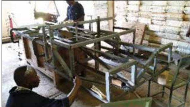
Figure 2. During frame fabrication.
